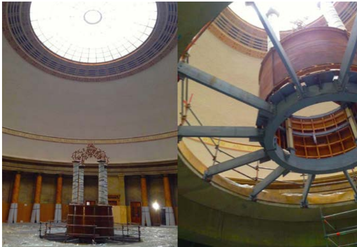
Figure 8 – Disassembling the dome room. Source: the Author.
