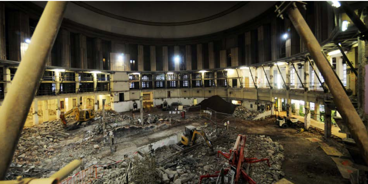
Figure 14 – Demolition during execution. Source: the Author.
